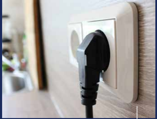
Socket type F is the Schuko socket. The Schuko plug is the most commonly used plug in Germany and Europe.
